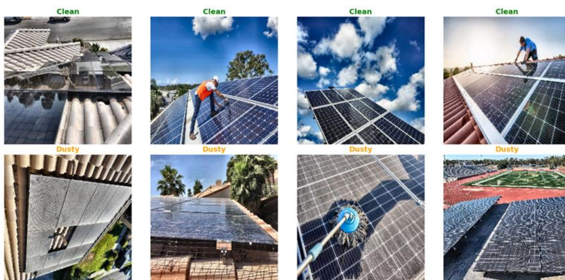
Figure 4: Sample training images illustrating clean and dust-affected photovoltaic panel surfaces
